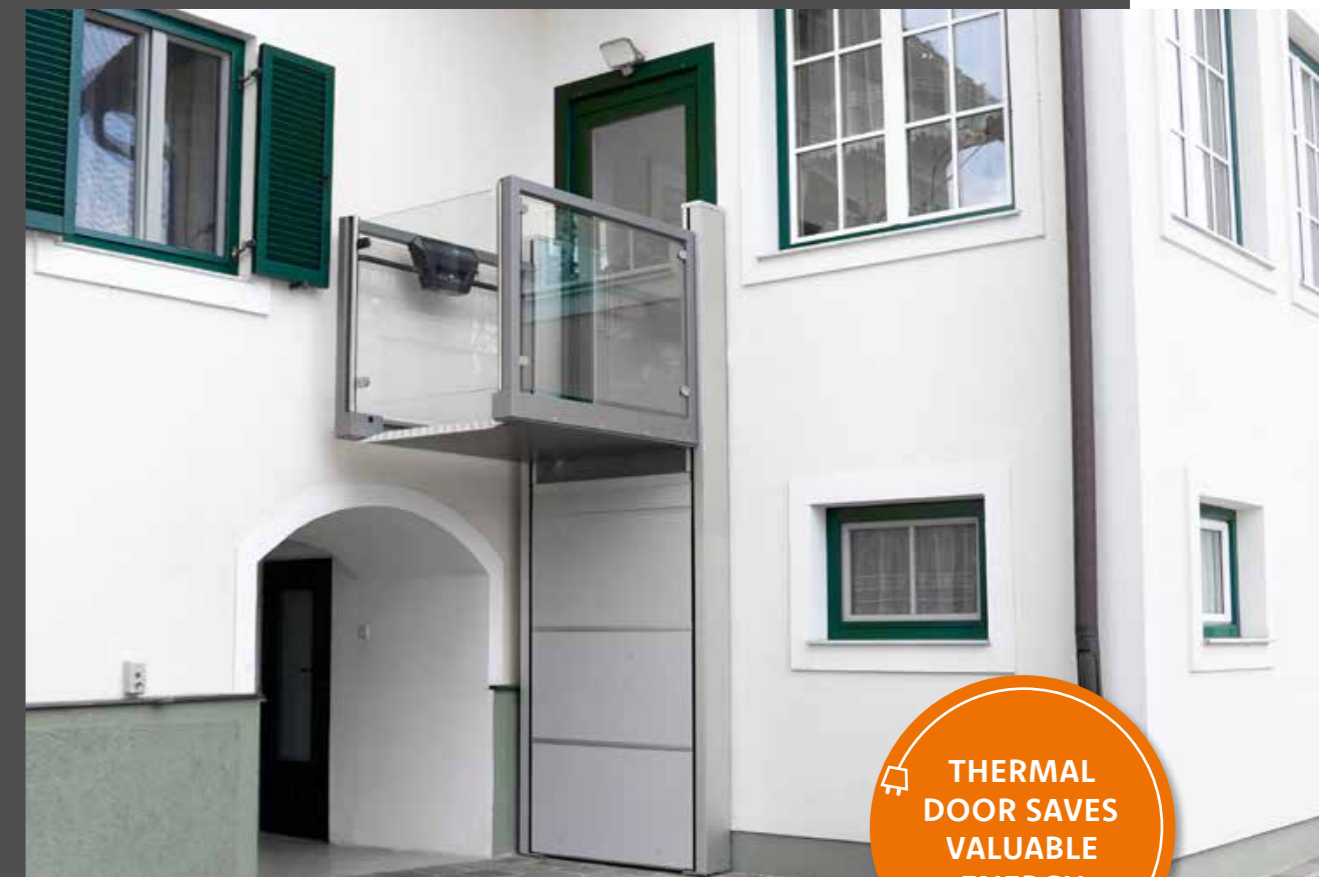
Easy retrofitting of a lift with thermal door.
